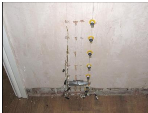
Figure 6 Multi-point moisture monitoring apparatus used for gravimetric assessment of a damp-affected wall
