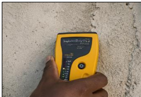
Figure 2 Electrical (Protimeter) moisture meter reading being taken on a masonry wall
